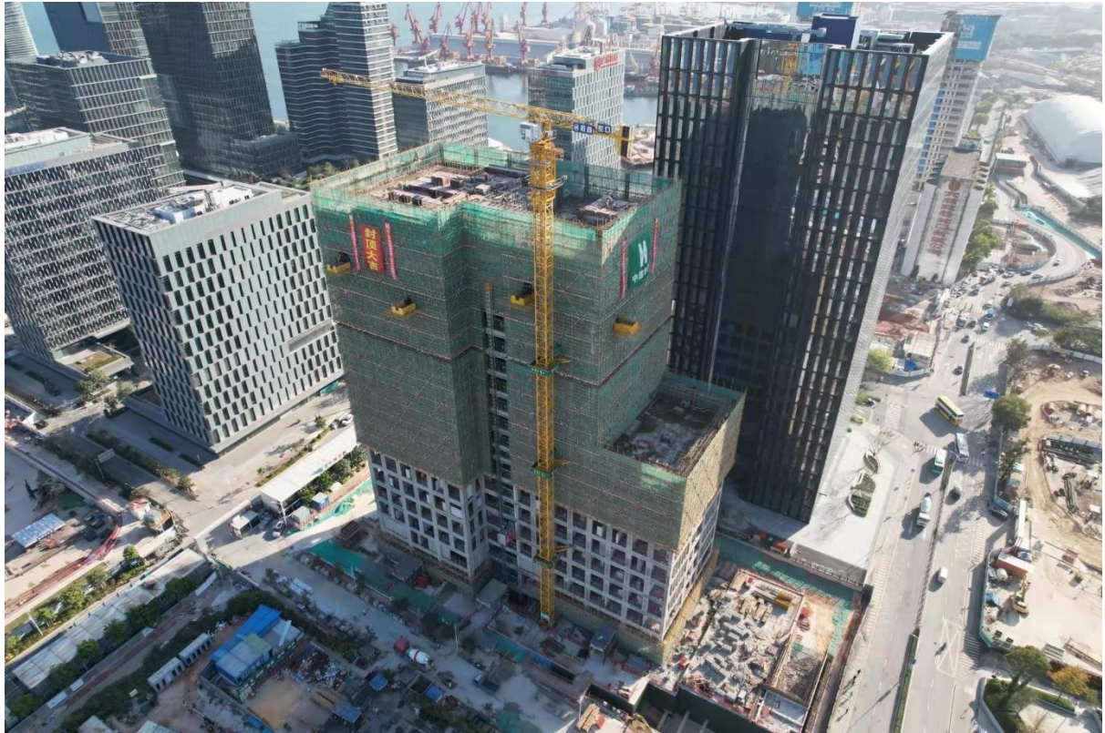
Prince Bay Hospital as at March 2022
